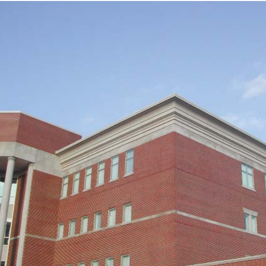
Michigan Catholic Conference Headquarters, Lansing, MI Wigen Tincknell Meyer & Assoc. Inc.
