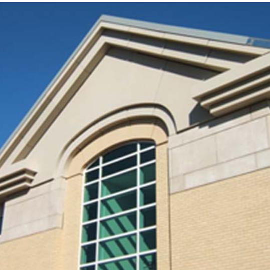
Clifton Park Halfmoon Public Library, Clifton Park, NY Woodward Connor Gillies Seleman Architects.
